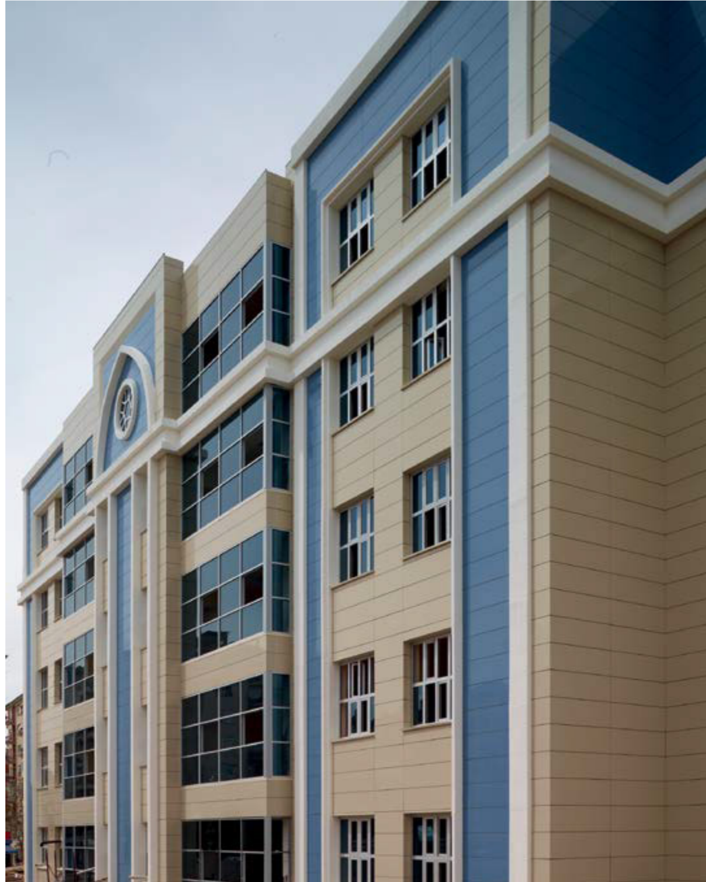
Adliye Sarayı / Kirsehir — NordicFlexBoard 5mm Fit Parlak Bej & NordicFlexBoard 5mm Fit Parlak Mavi / Gizli Klipsli Sistem Courthouse / Kirsehir — NordicFlexBoard 5mm Fit Polished Beige & NordicFlexBoard 5mm Fit Polished Blue / Hidden Clips Fitted Facade System Mimar : Sütichen Mimarlık — Architect : Sütichen Architectural Office
