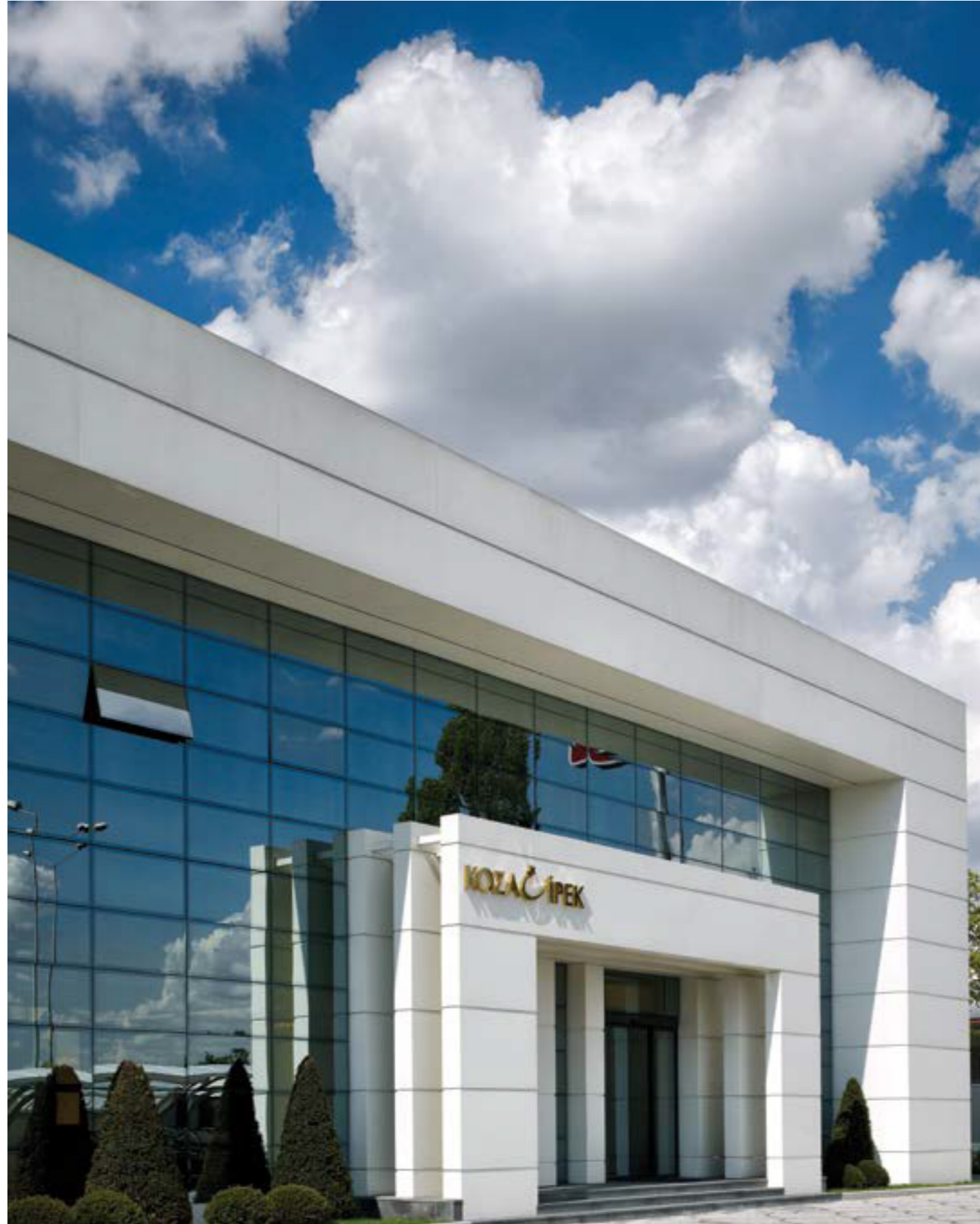
Koza Merkez Binası / Ankara / 100x300cm Düz Mega Beyaz Mat / Gizli Klipsli Sistem Koza Central Building / Ankara / 100x300cm Plain Mega White Matte / Hidden Clips Fitted Facade System Mimar : Promer Mimarlık — Architect : Promer Architectural Office
