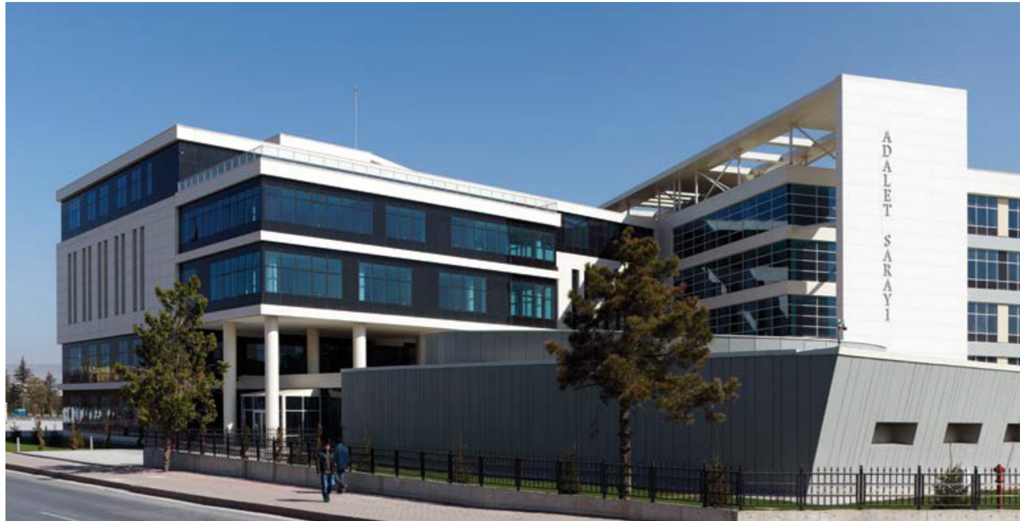
Kayseri Adliye Sarayı / Kayseri — 3mm Mat Fit Beyaz - 3mm Mat Fit Çimento Gri - 3mm Mat Fit Fildişi / Gizli Klipsli Sistem Kayseri Courthouse / Kayseri — 3mm Matte Fit White - 3mm Matte Fit Cement Grey - 3mm Matte Fit Ivory/ Hidden Clips Fitted Facade System Mimar : Ven Mimarlık — Architect : Ven Architects
