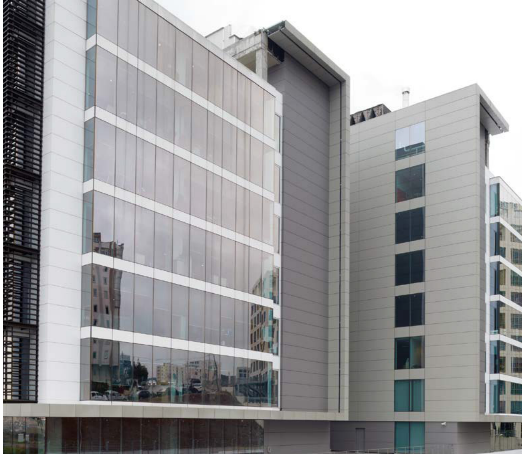
Kavacak İş Merkezi / İstanbul — 3mm Mat Fit Luxury Cement Gri - 3mm Mat Fit Antrasit / Gizli Klipsli Sistem Kavacak Business Center / İstanbul — 3mm Matte Fit Luxury Cement Grey - 3mm Matte Fit Anthracite / Hidden Clips Fitted Facade System Mimar : Cevahir İnşaat — Architect : Cevahir Construction Company
