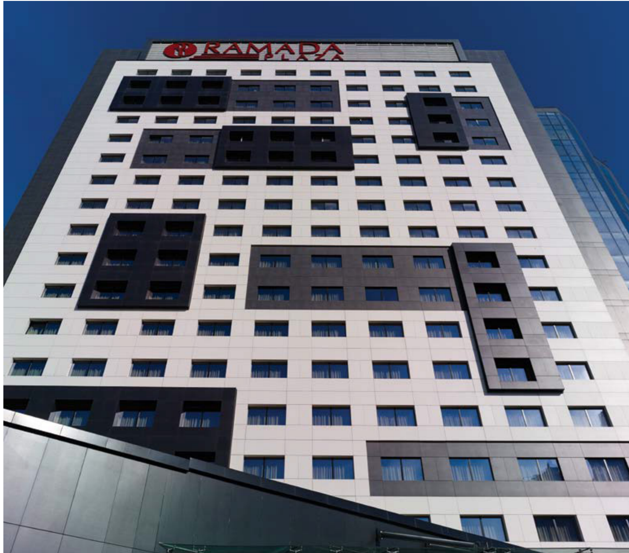
Ramada Plaza / İstanbul — 3mm Mat Fit Mega Siyah - 3mm Fit Mat Mega Beyaz - 3mm Mat Fit Luxury Cement Antrasit / Gizli Klipsli Sistem Ramada Plaza / İstanbul — 3mm Matte Fit Mega Black - 3mm Fit Matte Mega White - 3mm Matte Fit Luxury Cement Anthracite / Hidden Clips Fitted Facade System Mimar : M Ofis — Architect : M Office
