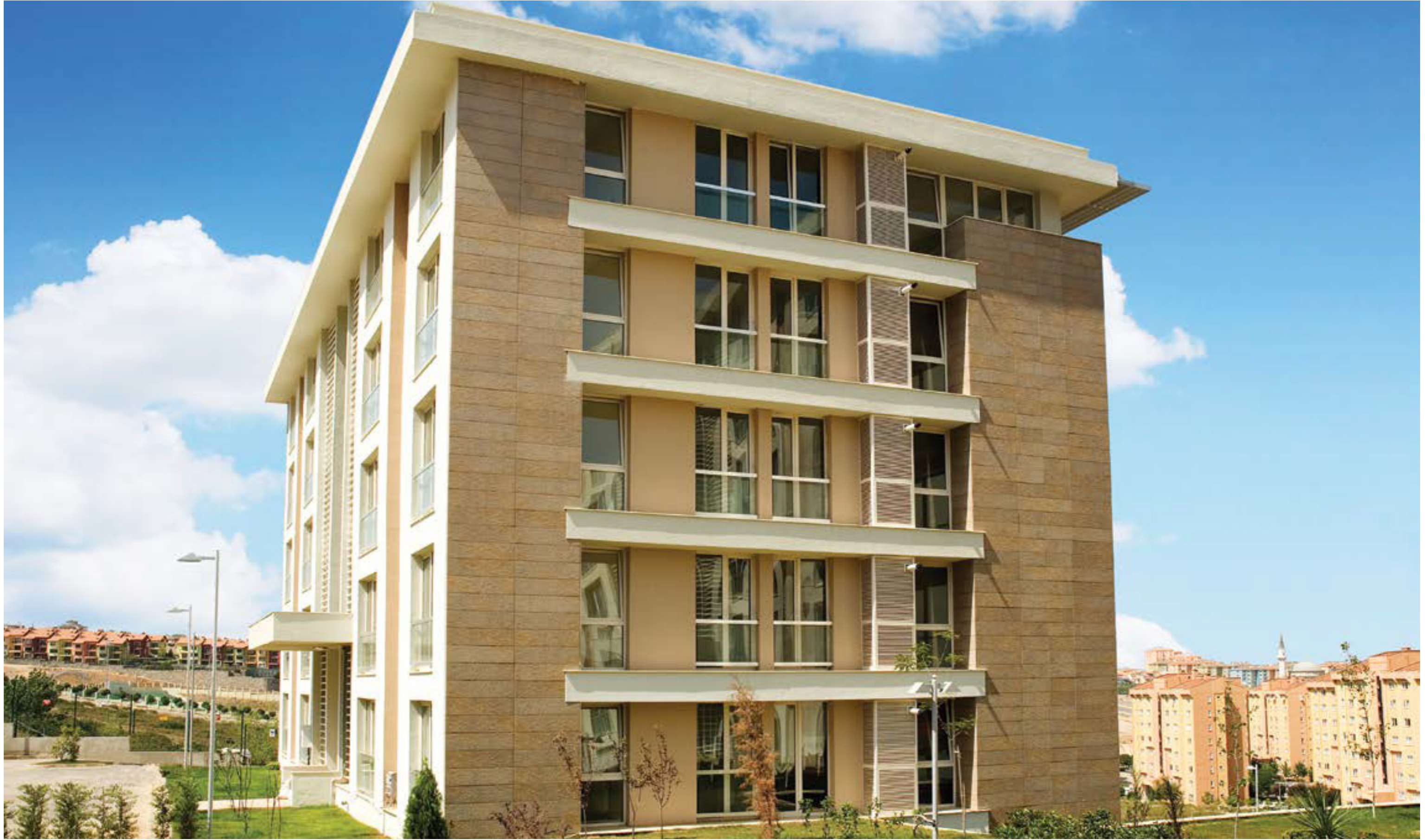
Crystal Park Konutları, Pendik / İstanbul — 30x120 Heraklia Stone Bej / Konstrüksiyona Yapıştırma Sistem Crystal Park Residence, Pendik / İstanbul — 12"x48" Heraklia Stone Beige / Adhesion System on Construction Mimar : Uras X Dilekçi Mimarlık — Architect : Uras X Dilekçi Architectural Office
