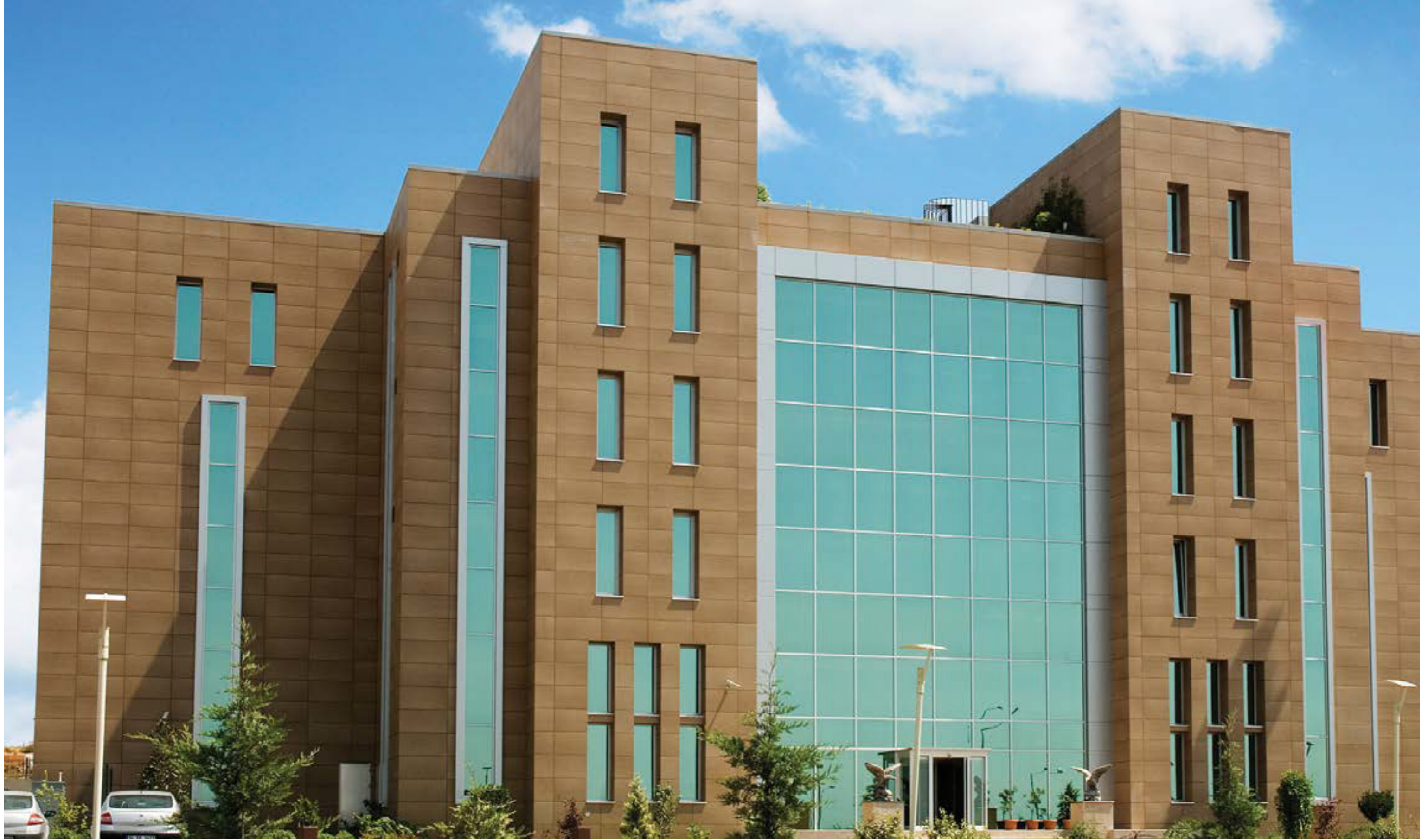
Oba Perde İdari Binası, Gebze / Kocaeli — 60x120 Apollon Stone Kahve / Klipsli Sistem Oba Perde Administration Office, Gebze / Kocaeli — 24"x48" Apollon Stone Brown / Clips System Mimar : Kapra İnşaat — Architect : Kapra Construction
