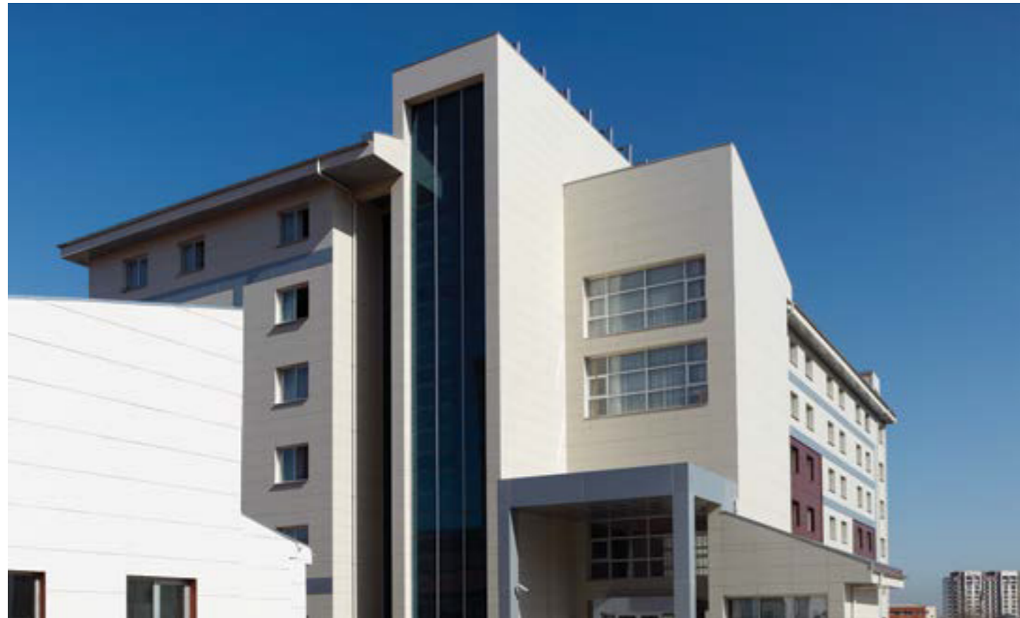
Kayseri 1000 Kişilik Bayındırlık Yurdu / Kayseri / 60x120cm Düz Beyaz Mat / Gizli Sistem Kayseri 1000-Person Public Works Dormitory/ Kayseri / 60x120cm Plain White Matte /Invisible System Mimar : Peb Mimarlık — Architect : Peb Architectural Office
