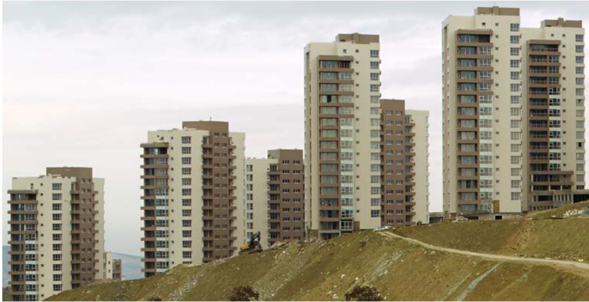
Toki İncek Konutları / Ankara — 3mm Mat Fit Beyaz - 3mm Mat Fit Bej Gri / Gizli Klipsli Sistem Toki İncek Residences / Ankara — 3mm Matte Fit White - 3mm Matte Fit Beige Grey / Hidden Clips Fitted Facade System Mimar : Nazan Sağlam Mimarlık — Architect : Nazan Sağlam Architects
