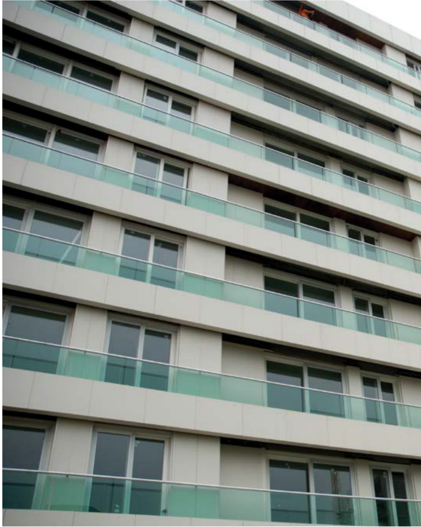
Novus Residence, Ataköy / İstanbul — NordicFlexBoard 3mm Fit Beyaz / Gizli Klipsli Sistem Novus Residence, Ataköy / İstanbul — NordicFlexBoard 3mm Fit White / Hidden Clips Fitted Facade System Mimar : TAGO Mimarlık — Architect : TAGO Architectural Office
