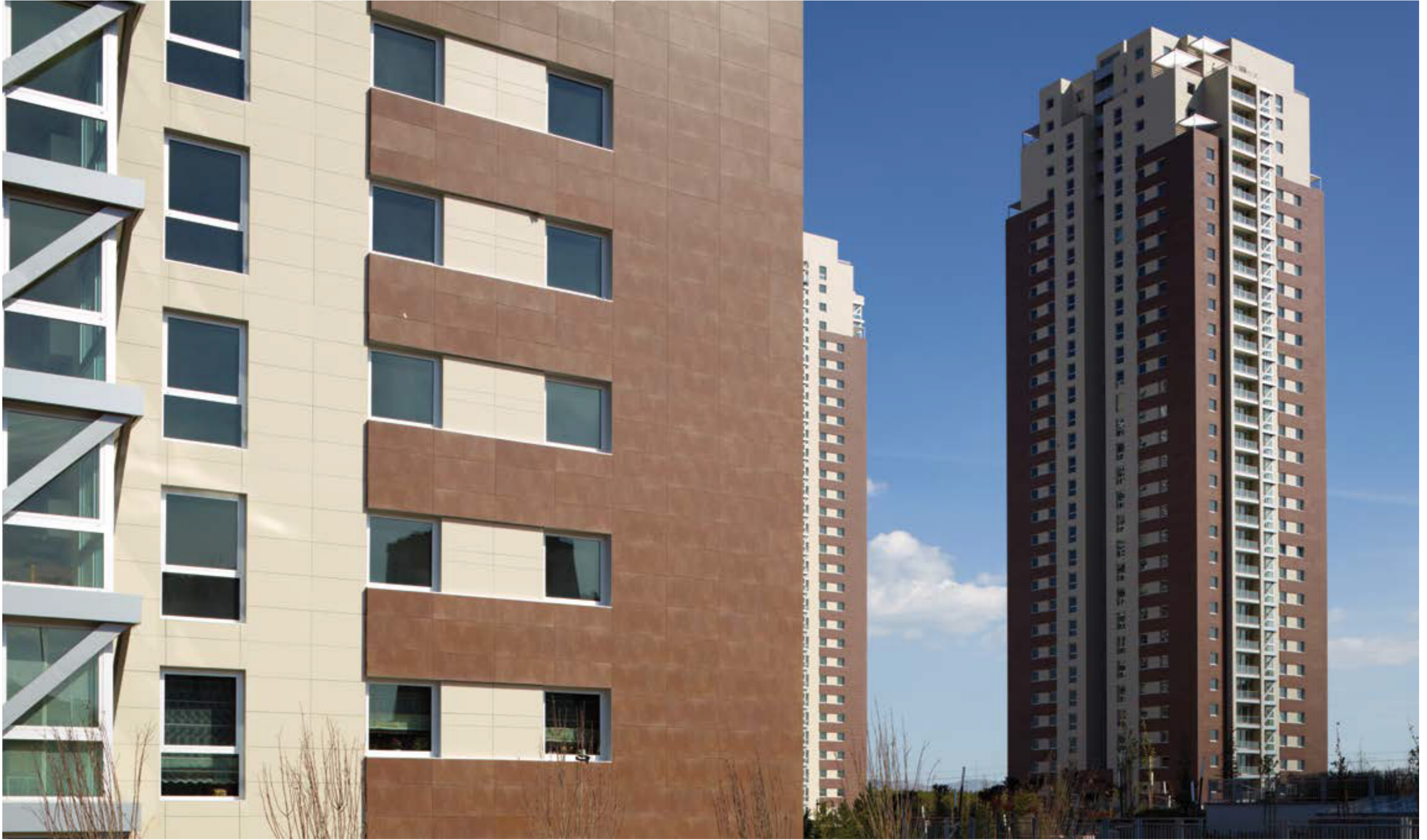
Mesa Park Oran Konutları / Ankara — 60x120 Luxury Cement Kahve & 60x120 Düz Bej Mat / Gizli Sistem Mesa Park Oran Residence / Ankara — 24"x48" Luxury Cement Brown & 24"x48" Plain Beige Matte / Invisible System Mimar : ACE Mimarlık — Architect : ACE Architectural Office
