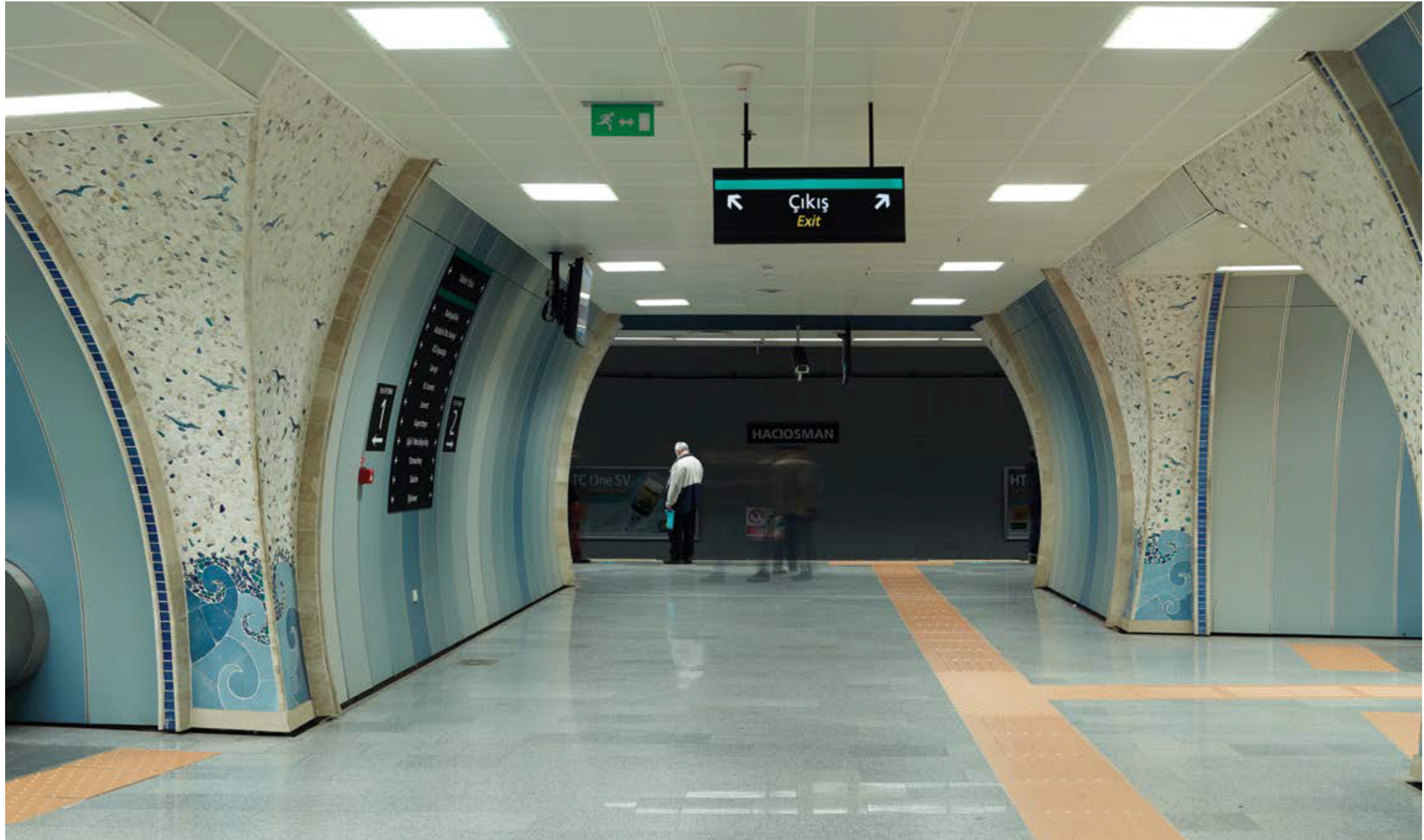
Haciosman Metro Durađı / İstanbul — 3mm Fit Mat Özel Renk Çalıřması Haciosman Metro Station / İstanbul — 3mm Fit Matte Special Color Mimar : Yüksel Proje — Architect : Yüksel Project
