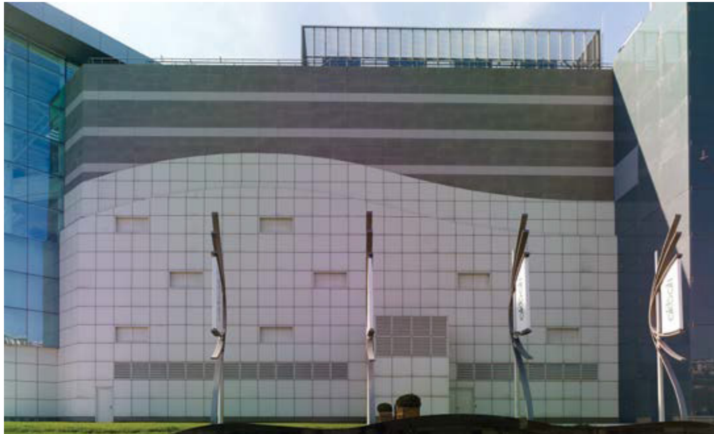
Akbatı AVM, Esenyunt / İstanbul — 60x120cm Heraklia Stone Beyaz - 60x120cm Apollon Stone Yeşil / Klipsli Sistem Akbatı AVM, Esenyunt / İstanbul — 24"x48" Heraklia Stone White - 24"x48" Apollon Stone Green / Clips System Mimar : Seçkin Mimarlık — Architect : Seçkin Architectural Office
