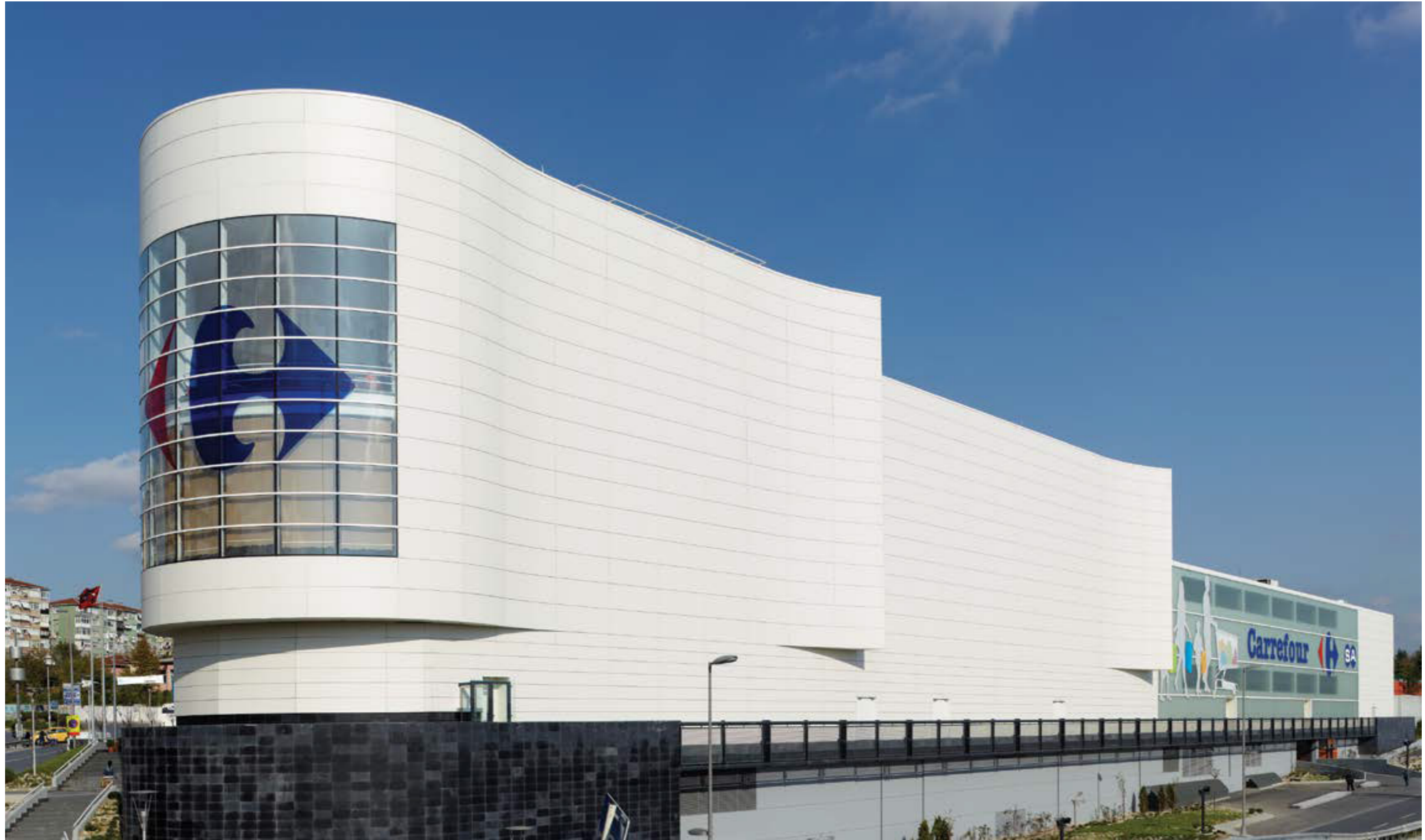
Carrefour AVM, Bahçelievler / İstanbul — NordicFlexBoard 3mm Fit Beyaz / Gizli Klipsli Sistem Carrefour AVM, Bahçelievler / İstanbul — NordicFlexBoard 3mm Fit White / Hidden Clips Fitted Facade System Mimar : Era Mimarlık — Architect : Era Architectural Office
