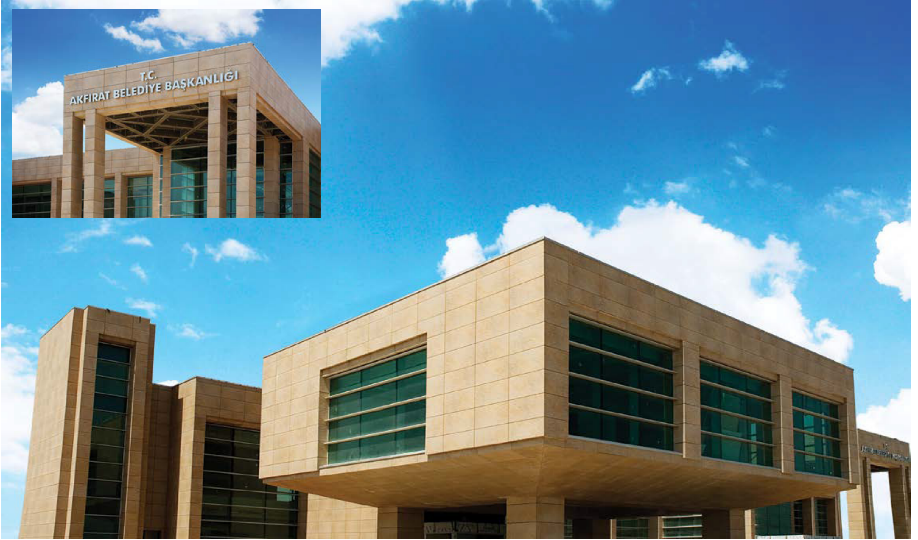
Akfırat Kültür Merkezi, Tuzla / İstanbul — 60x120 Heraklia Stone Bej / Gizli Sistem Akfırat Cultural Center, Tuzla / İstanbul — 24"x48" Heraklia Stone Beige / Invisible System Mimar : Geyran Mimarlık — Architect : Geyran Architectural Office
