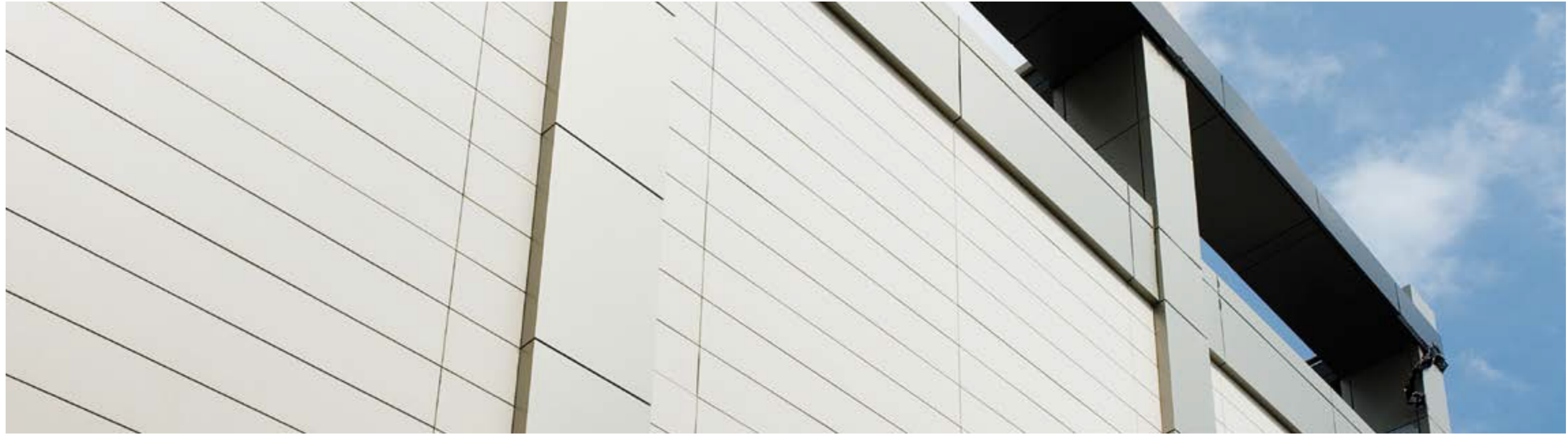
Bakırköy Capacity Alışveriş Merkezi / İstanbul — NordicFlexBoard 3mm Fit Bej / Gizli Klipsli Sistem Bakırköy Capacity Mall / İstanbul — NordicFlexBoard 3mm Fit Beige / Hidden Clips Fitted Facade System Mimar : Konsept Mimarlık — Architect : Konsept Architectural Office
