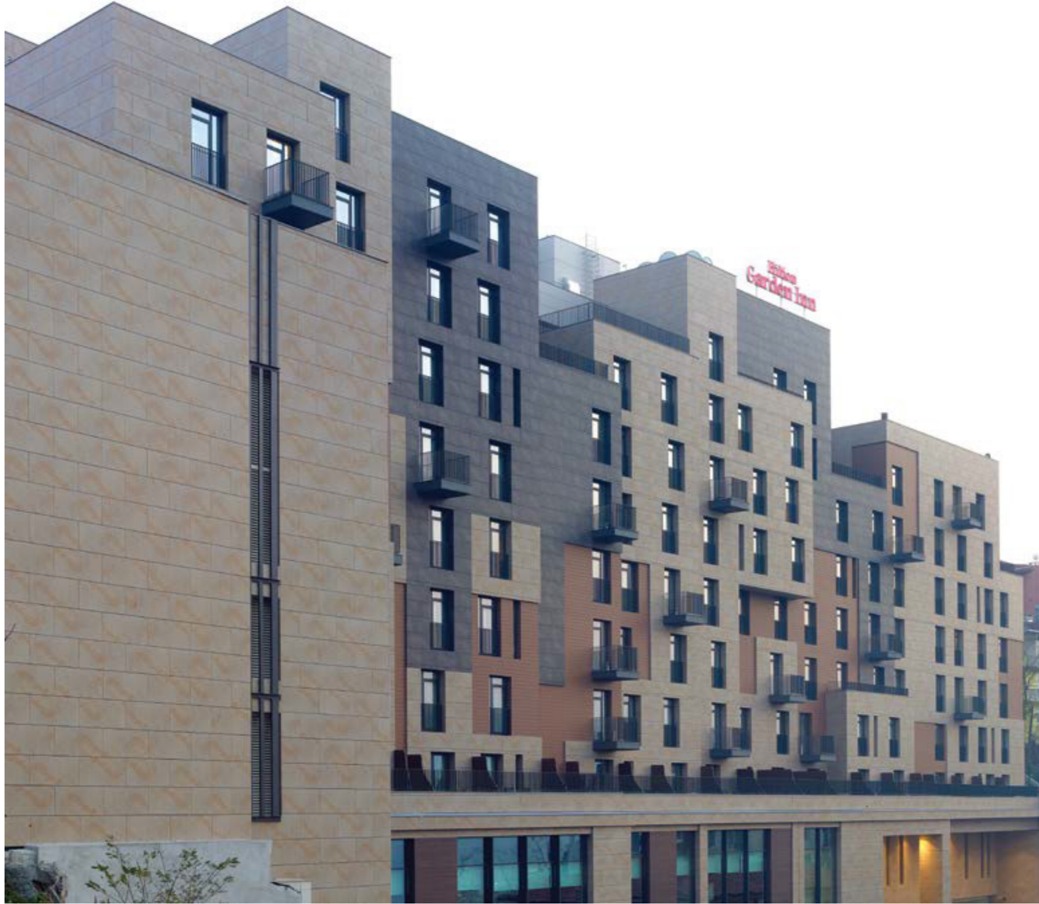
Hilton Garden Inn İstanbul Golden Horn / İstanbul — Heraklia Stone Bej - Heraklia Stone Koyu Gri 60x120cm / Gizli Sistem Hilton Garden Inn İstanbul Golden Horn / İstanbul — Heraklia Stone Beige - Heraklia Stone Dark Grey 24"x48" / Invisible System Mimar : TeCe Mimarlık — Architect : TeCe Architectural Office
